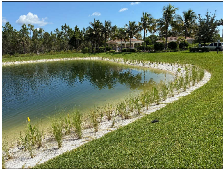
Figure 1. Vegetated Regraded Lake Bank. (Seabreeze Erosion Solutions, 2025)
